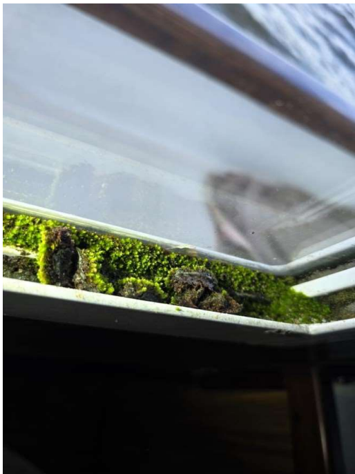
Grime/mildew buildup in window tracks
