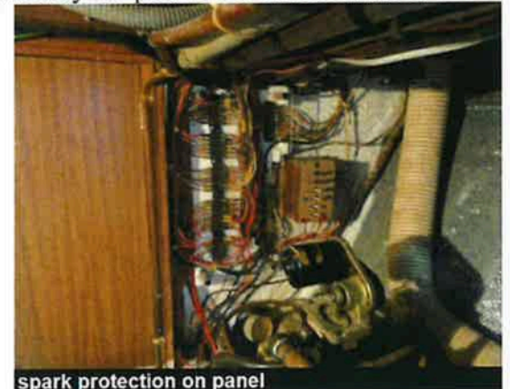
spark protection on panel
